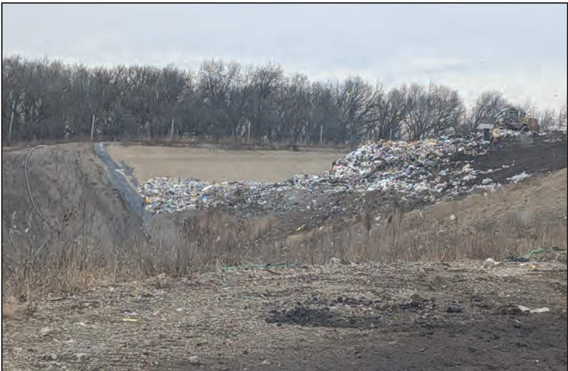
Working face in Northwest corner, deep fill
