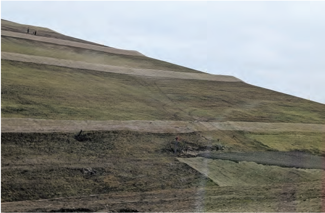
West slope of capping project
