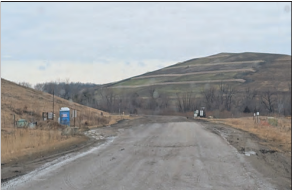
Capping project weathering nicely
