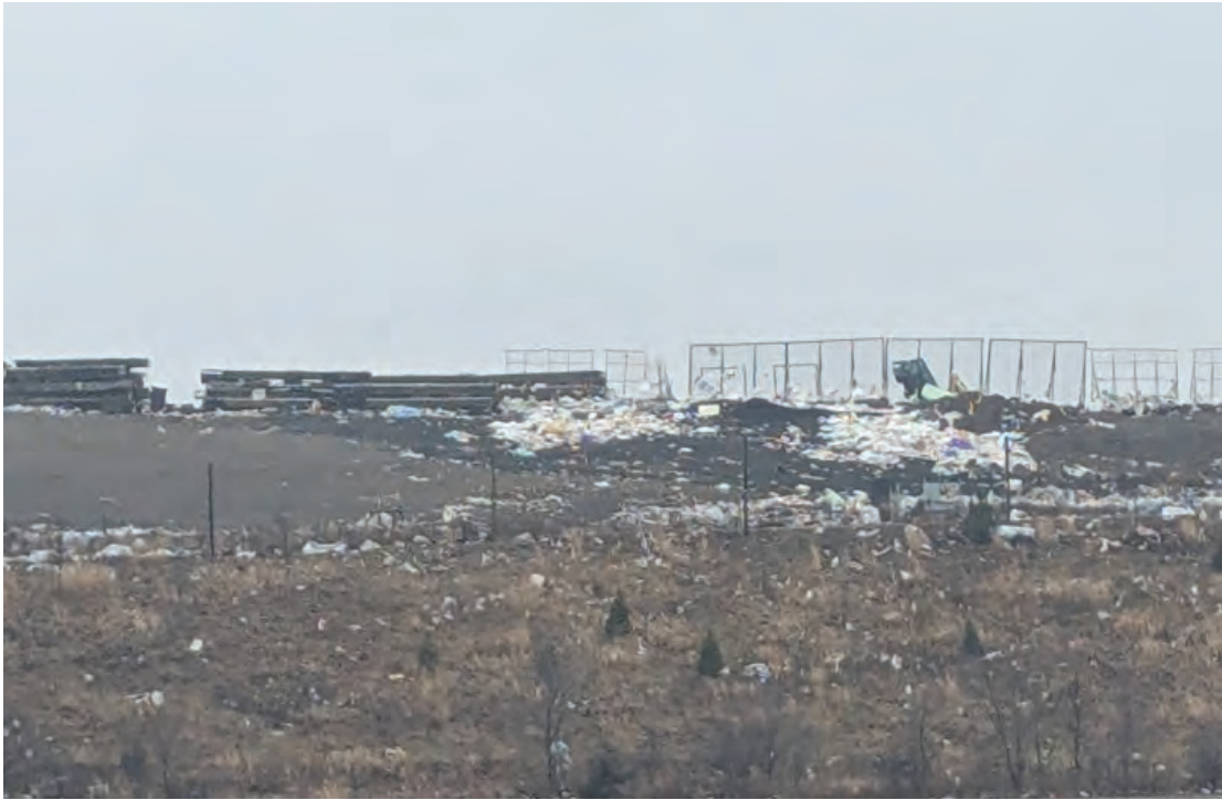
Phase 4 viewed from South - note gap in fences allowed litter to accumulate
